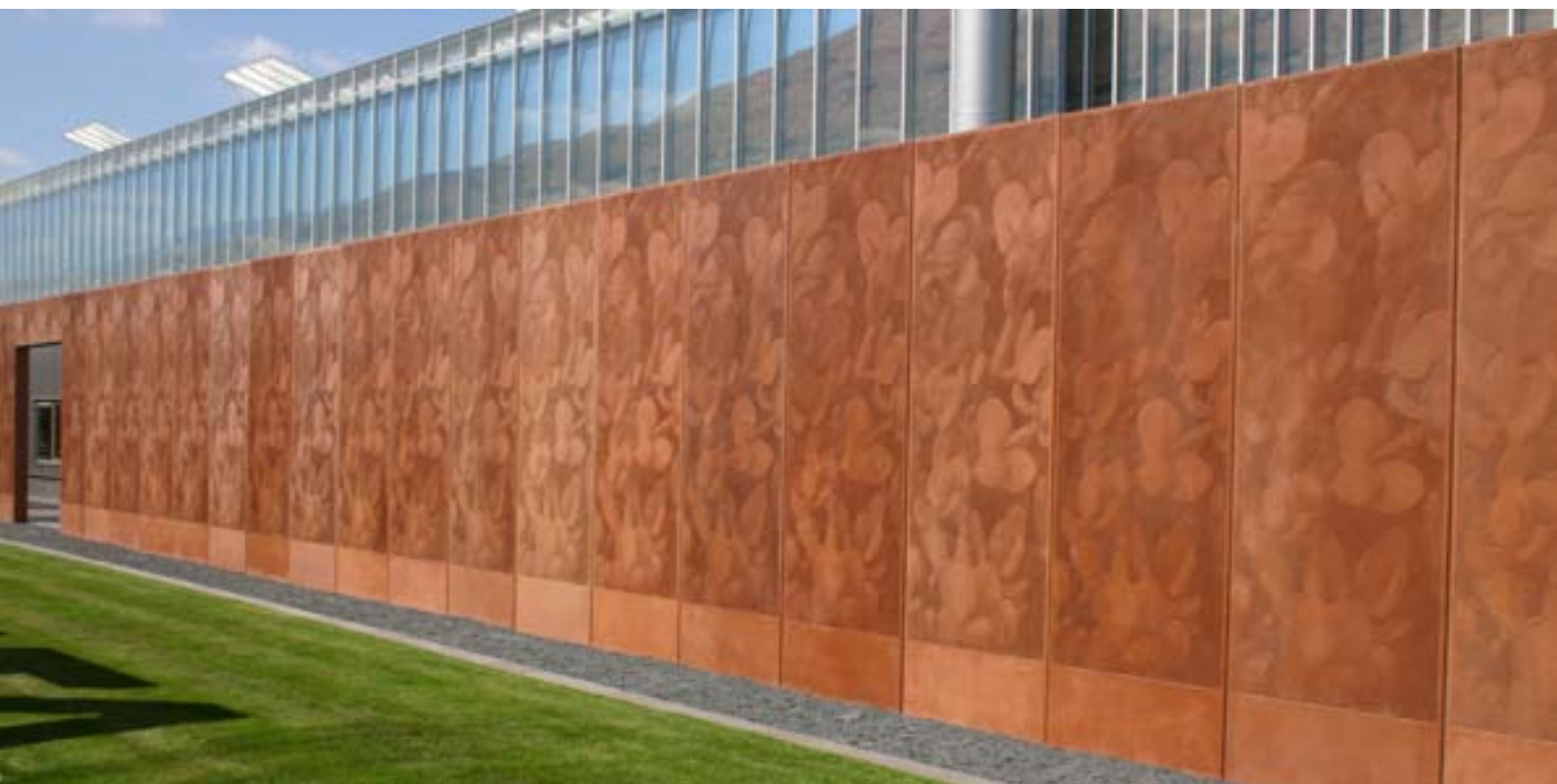
From photo to precast part: original photo master, formliner and concrete element with photo-engraved motif.
